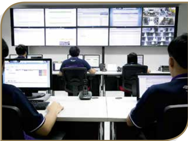
Network Operation Center (NOC)
